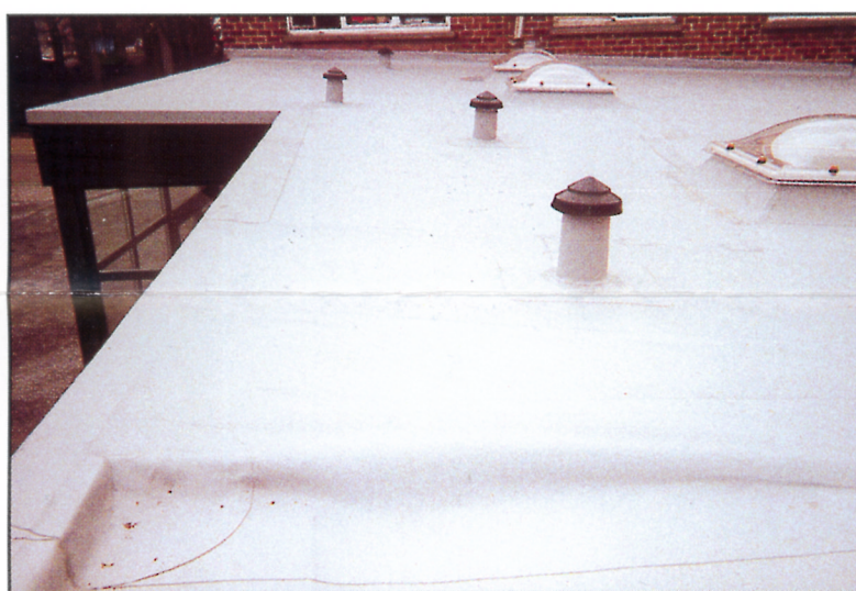
Sintofoil on BMB's roof
