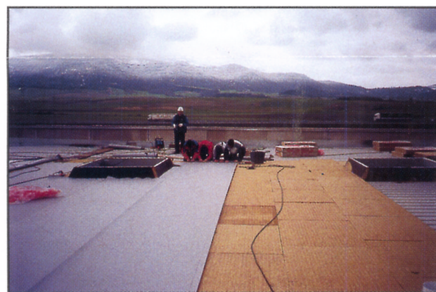
Pulling ST membrane before fixing.
