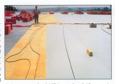
took no chance: Rubberfuse mechanically attached system, using Sintofoil ST (non reinforced) 1.2mm was the obvious choice. The combination of the performing, competitive FPA membrane with a fast, easy to install system, resulted in a trouble-free, on-time installation. Notes for the record: Acieroid are pioneers, as they completed, in 1994, one of the first FPA projects in Europe and Acieroïd's prestigious references list includes the 60.000m² Coca Cola bottling plant located in Seville.
