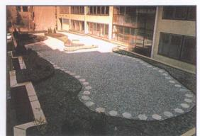
Environment is a growing concern. This explains the success of "green roofs". Such system provides a pleasant, colourfull touch to the 400m2 terrace of the MTA-STZAKI Headquarters. Sintofoil resists to puncture and root penetration. The ST type membrane was loose-laid, to provide optimal flexibility for the system.
