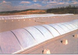
Fast track project usually implies quick installation. This is why a mechanically attached single-ply system was selected for the new 5.200m2 OBI Shopping Center. As the structure is a light steeldeck, the membrane will have to cope with permanent substrate movements. The long-term performance as offered by Sintofoil is the appropriate answer: the FPA membrane is inert, ie will remain flexible throughout the years. As aesthetics were also a concern, the reinforced grey membrane was selected.
