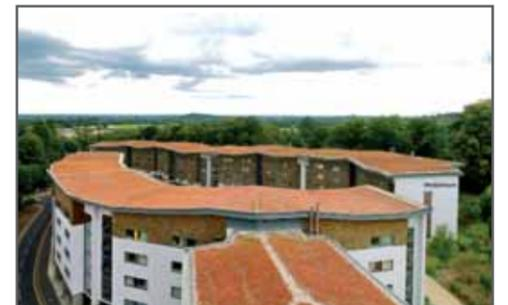
The new extension of students accommodations is covered by a Rubberfuse green roof. The build up is concrete deck, vapour barrier, 90mm PIR insulation, Sintofoil membrane, drainage mat, filter layer and sedum greening layer. The sedum is composed of many varieties of seeds, chosen by an expert horticulturist to best suit the environment and conditions.
