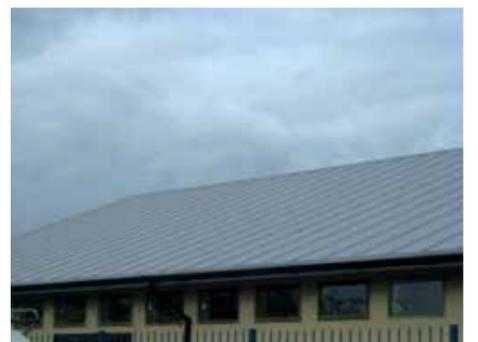
The building is intended to be used for not more than 5 years, however the designer stipulated that all components should last 15 years or more. The Sintofoil membrane was selected as a non PVC environmentally sensitive material which could be recycled post use. It had to be aesthetically pleasing and be able to mimic the more expansive standing seam metal roof. The FB Sintofoil membrane was fully adhered system to eliminate any possible wrinkles.
