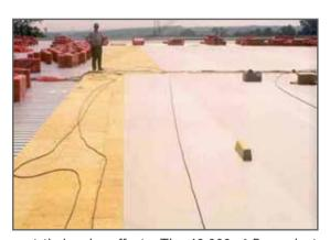
already available to support their sales efforts. The 40.000m² Roca plant in Gliwice, an export project carried out by Acieroid (Spain) has a Rubberfuse roof using Sintofoil ST mechanically attached on steel deck and Rockwool insulation. The initial phase was installed in 1997 and an extension has been recently completed.
