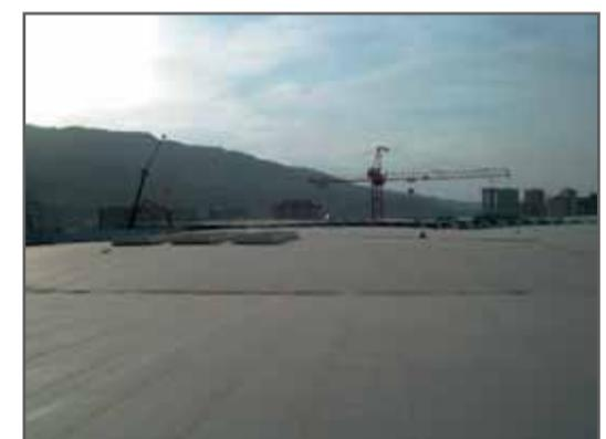
The Rubberfuse system was selected for its long-term performance (there are references exceeding 10 years in Spain), aesthetics and fire resistance (the system meets the ENV1187:2003 European requirement). The membrane is mechanically secured using Rubberfuse standard fixings (M-45 polyamide "locking" plate and BS 5,5 fastener). The building is not far away from the coast, so the wind uplift calculation led to using 1.05m wide sheets.
