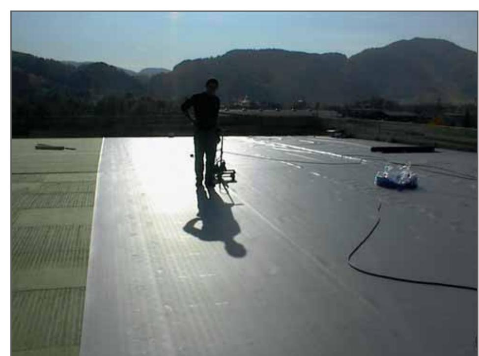
A few minutes later, after a short explanation and adjustments at the welding machine, the works resume. And all the trouble is a thing of the past. The picture tells it all... and proves the point: TPO/FPA is not « just another membrane ». Preliminary training is a prerequisite to get the job properly done.
