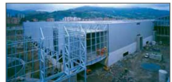
Acieroid won the turnkey contract for the entire envelope (roofing and cladding). The roof includes a perforated steel deck, which is lined with a special geotextile for optimal sound absorption. The insulation is 50mm thick Eurothane's Powerdeck and the membrane is TPO/FPA Sintofoil ST/FR1/Grey 1.2mm thick.
