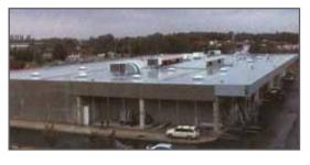
contacts with Ravago, Mrs Jelka Solmayer, the Architect in charge for this 4.000m<sup>2</sup> supermarket, decided to specify TPO/FPA. Sintofoil ST was selected, as let alone outstanding weathering performances, the membrane is totally environmentally friendly. Sintofoil was mechanically secured on the substrate (prefab concrete and 160mm thick Rockwool insulation). SCT, a well established applicator based in Ljubljana, successfully completed the roofing contract in July.
