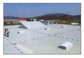
tem is Sintofoil ST on 160mm insulation and 0.7mm steel deck mechanically attached with Thermal Shut Rubberfuse fixings.
